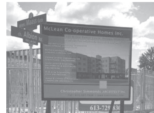
McLean Co-op under construction
